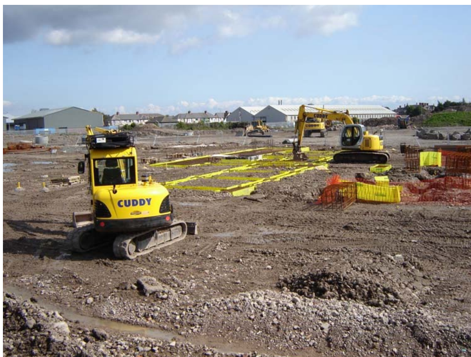
Site preparations, September 2008
